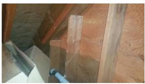
The framing is 2" x 6" wood members. The visible portions of the walls are framed with Framing members sizing.
