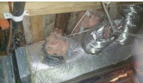
Duct Insulation in Unheated Exposed ductwork in unheated spaces is insulated adding to the efficiency of the Spaces: heating and air conditioning systems.
