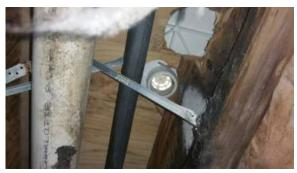
Vent Piping Material The vent material, as it passes through the roof, is plastic.
