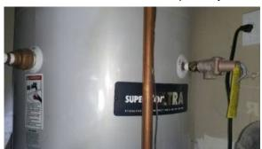
Water Piping Condition: Satisfactory - The incoming and output piping is installed correctly.
